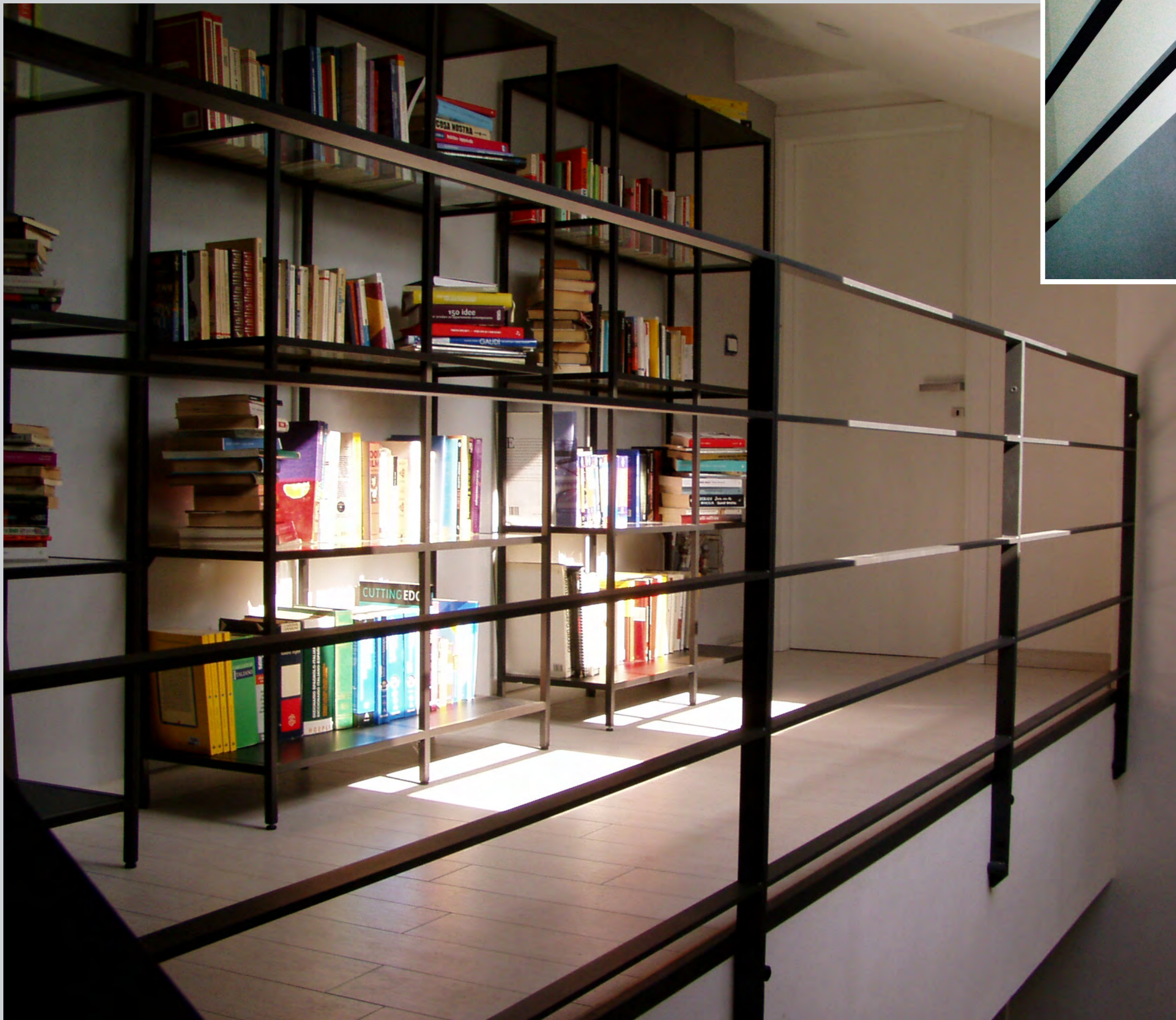
Balaustra DANAЕ, in ferro verniciato nero DANAЕ balustrade, made of black painted iron
